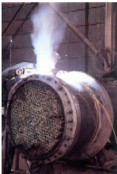
Heat exchanger repair.
